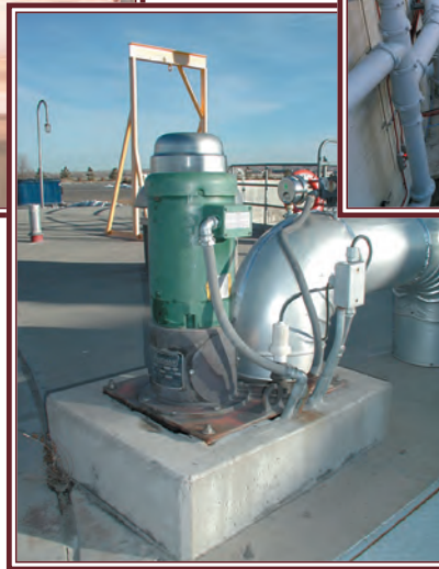
Primary Clarifier Scum
